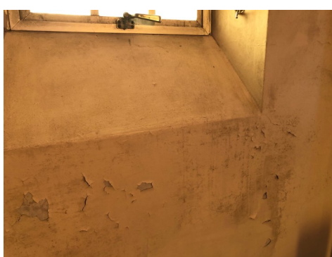
The dual issue: mould and peeling paint ↑
